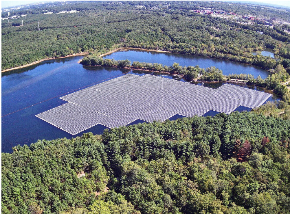
Floating solar array Sayreville, NJ, Water Authority 11 acres, 4.4 MW Second largest floating array in US
